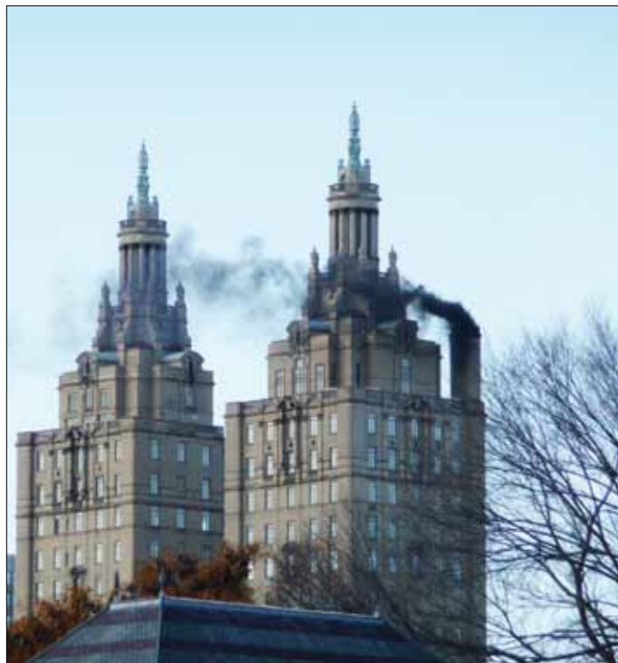
San Remo building burning No. 6 heating oil.
